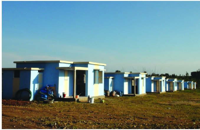
Newly constructed houses for villagers; (below) a family poses in front of its harvest
